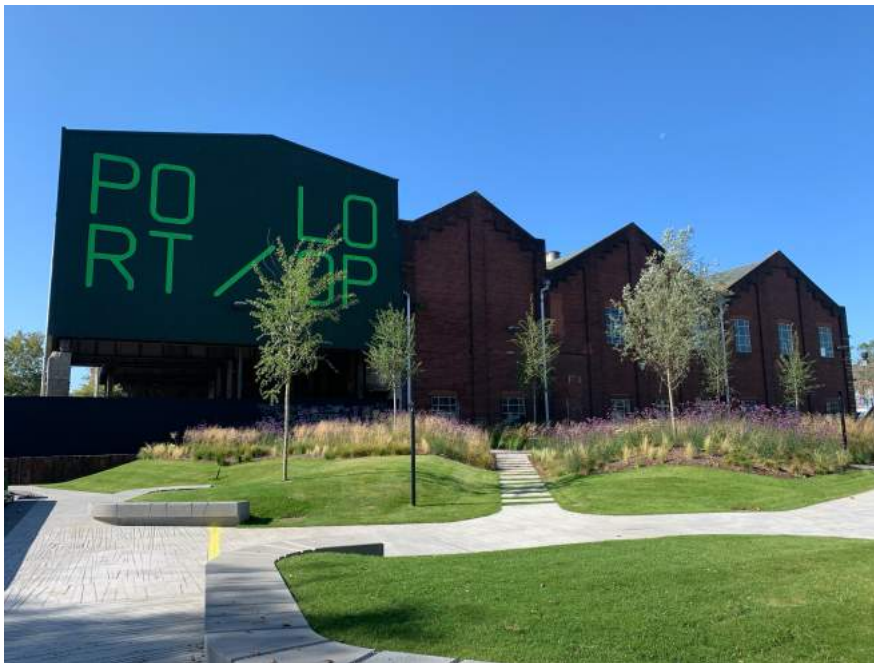
Figure 5: Image of original buildings being retained to house the Tubeworks.
